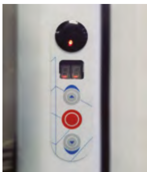
External pushbutton panel with touchless system
