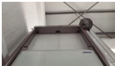
Detail of third safety cable.
