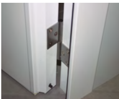
Guillotine weather strip integrated into leaf
