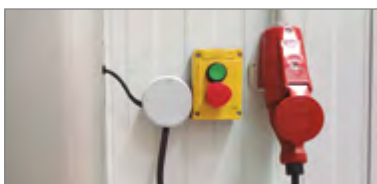
Interior safety button suitable for low temperature (provided as standard).
