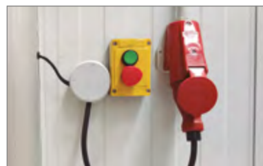
Indoor safety button panel adapted to low temperature (supplied as standard)
