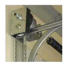
With chain hoist – good for doors with height more than 3m
