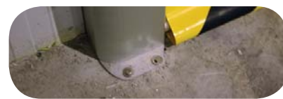
Fixed to the floor
